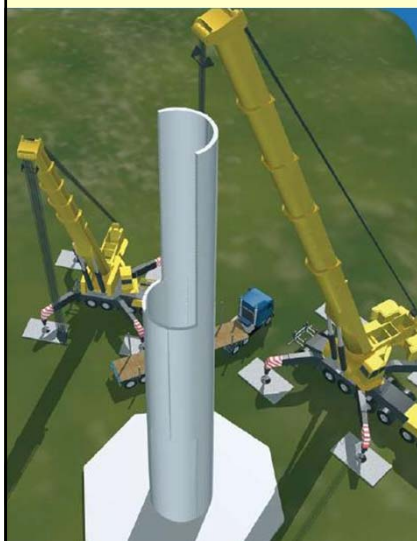
Figure 1: Typical precast concrete configuration
